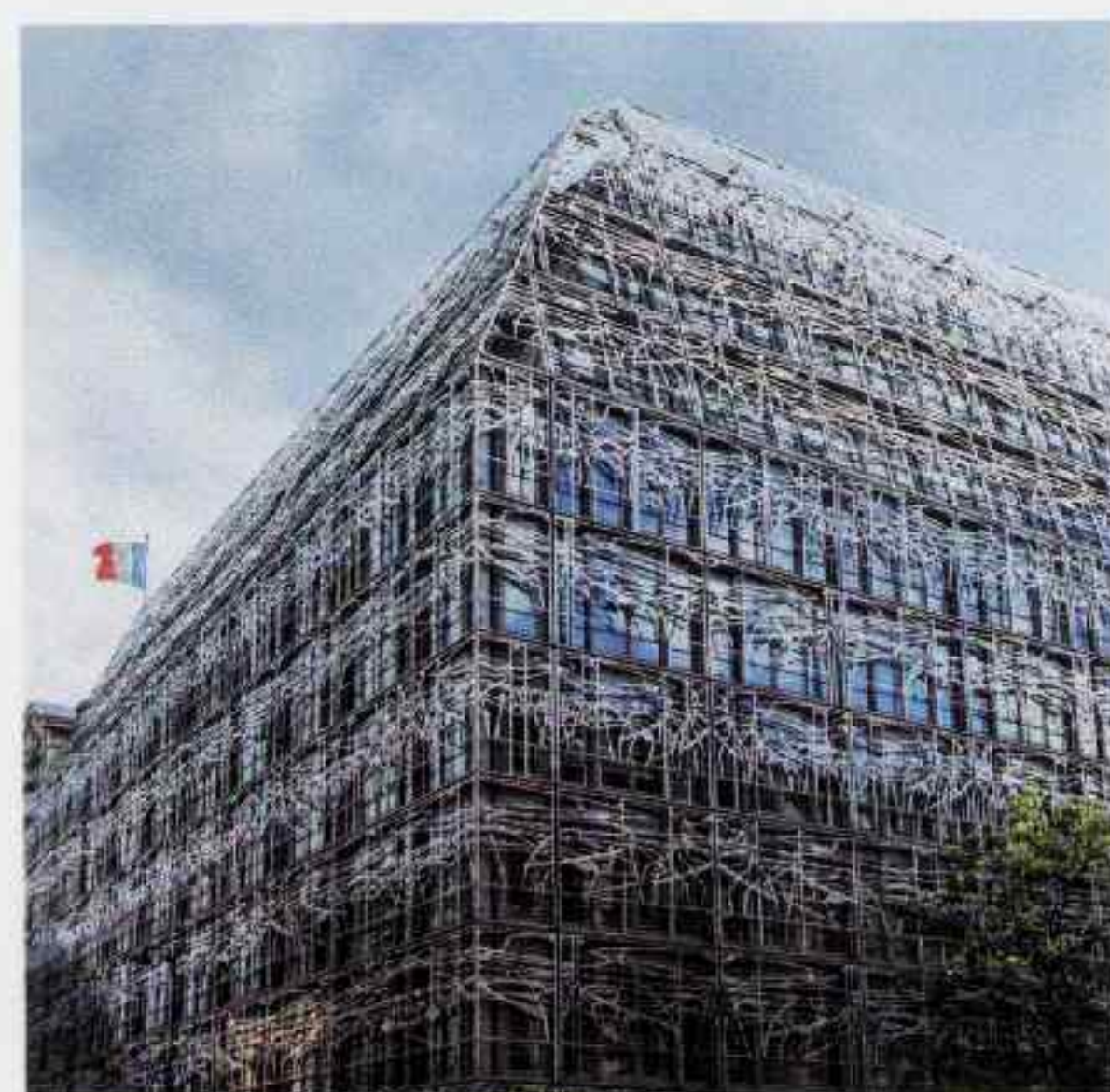
Suprafața ca ornament. Clădirea Ministerului Culturii, Paris, 2002-2004, arhitect Francis Soler Surface as ornament. The building of the Ministry of Culture, Paris, 2002-2004, architect Francis Soler
